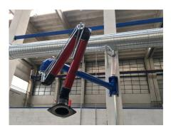
Welded steelextension with wall bracket for wall-mounted suction arms.
