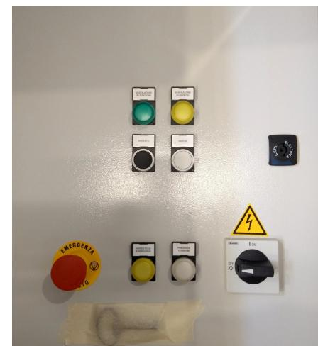
Direct-start and star-delta **industrial switchboard** for starting and protecting fan motors with 3F+T 400Vac 50/60Hz power supply.
